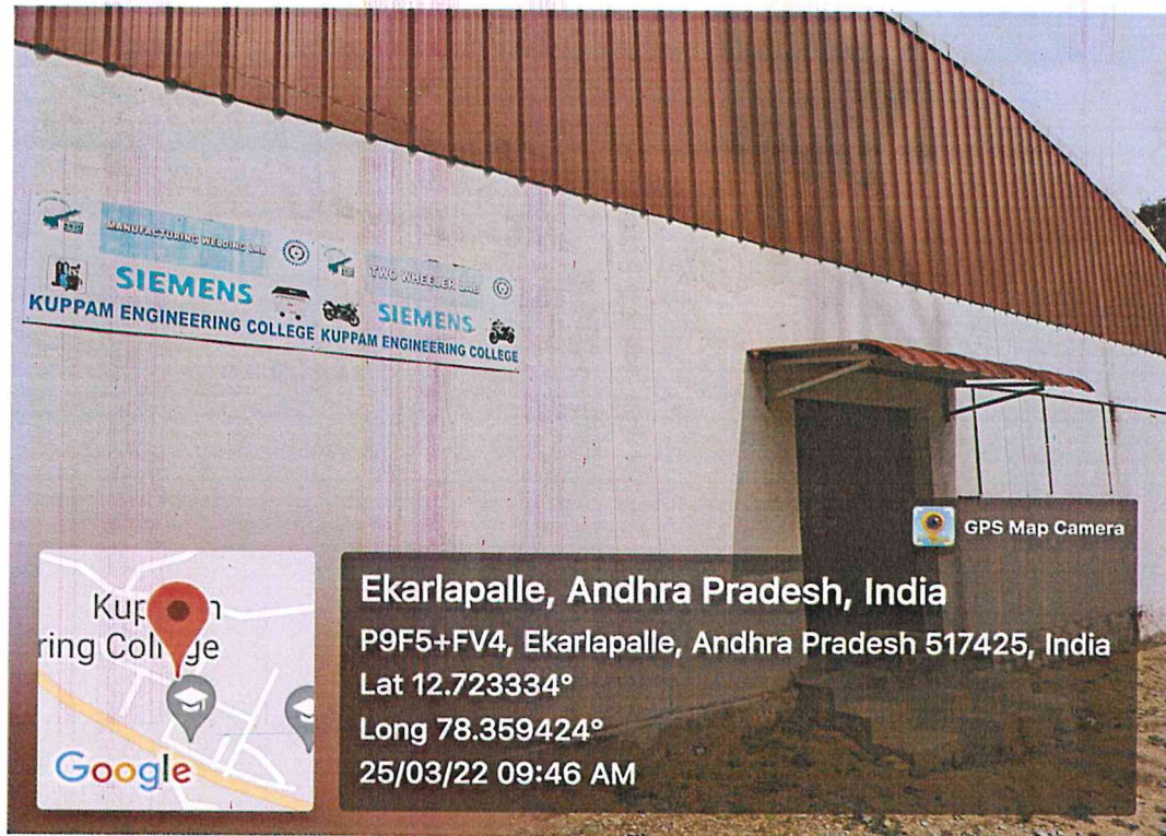
JRD TATA BLOCK (SIEMENS LABS)
